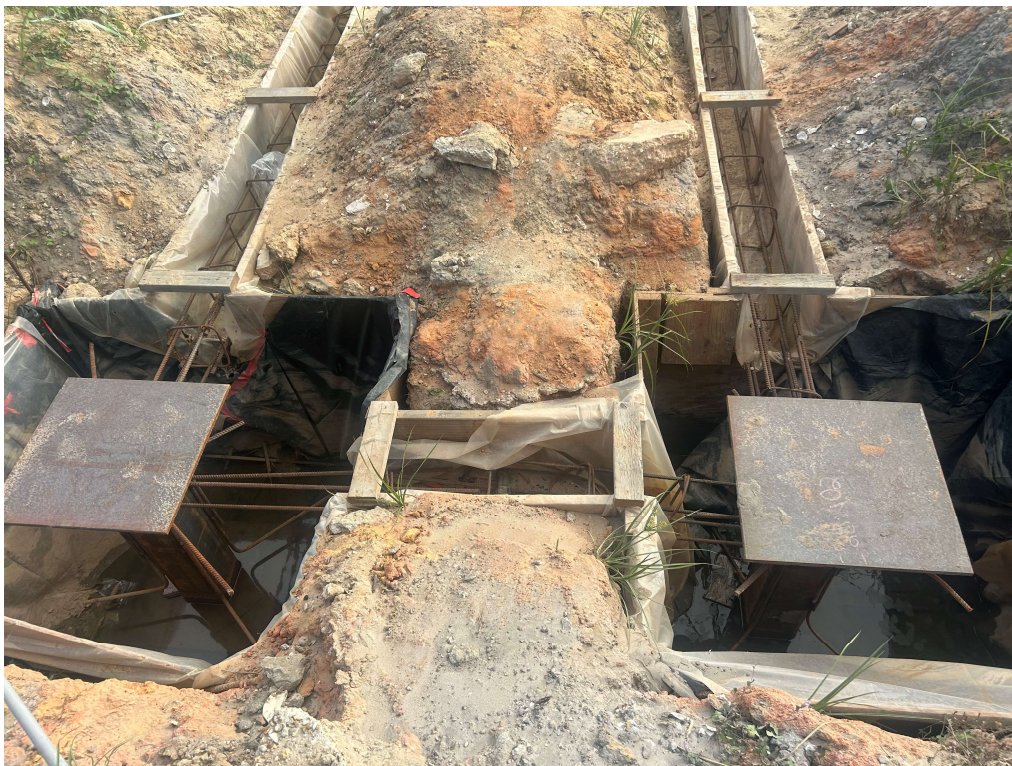
View of top of large footing under pool column showing embedded plate pedestal and grade beams
