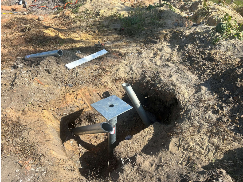
View of top of helical pile shafts with proprietary top plate for connection to columns
