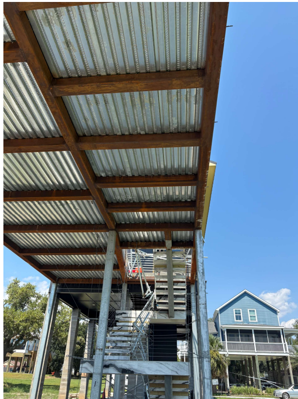
View of Structural Decking showing columns, beams and concrete deck pan
