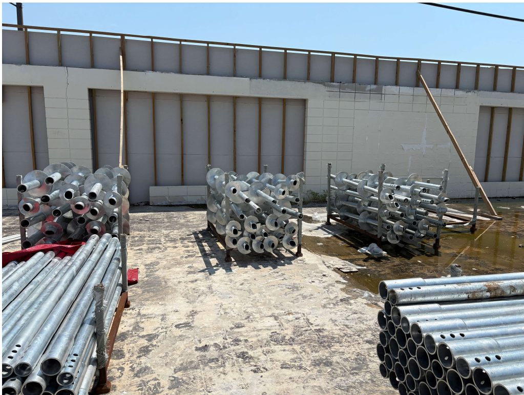
View of helical piles and shafts at the Bohn St warehouse
