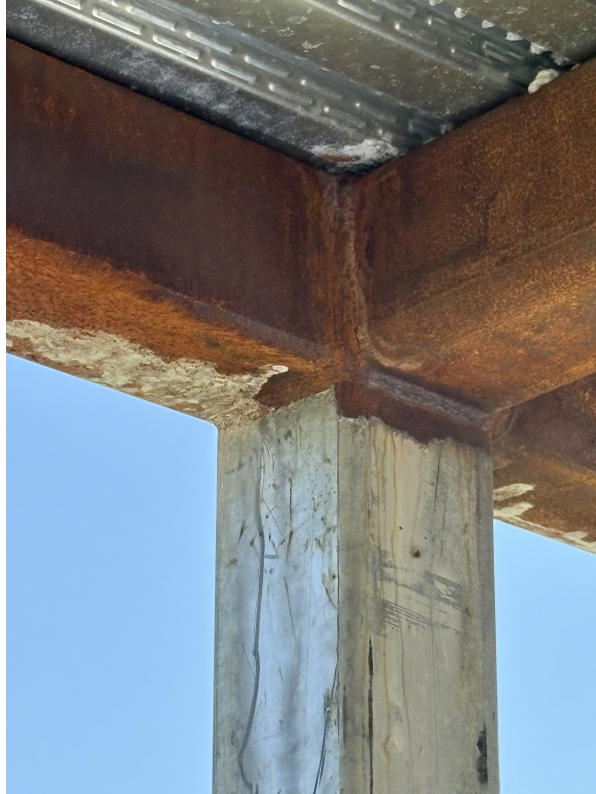
View of Structural connection at columns to beams denoting a moment frame
