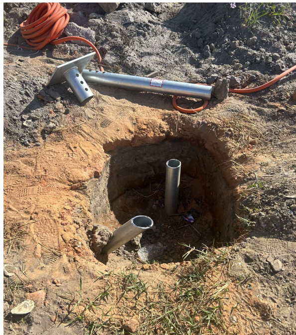
View of top of helical pile shafts. Vertical and batter pile shafts shown
