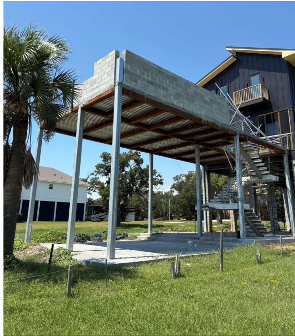
Front or south elevation showing the structural pool deck
